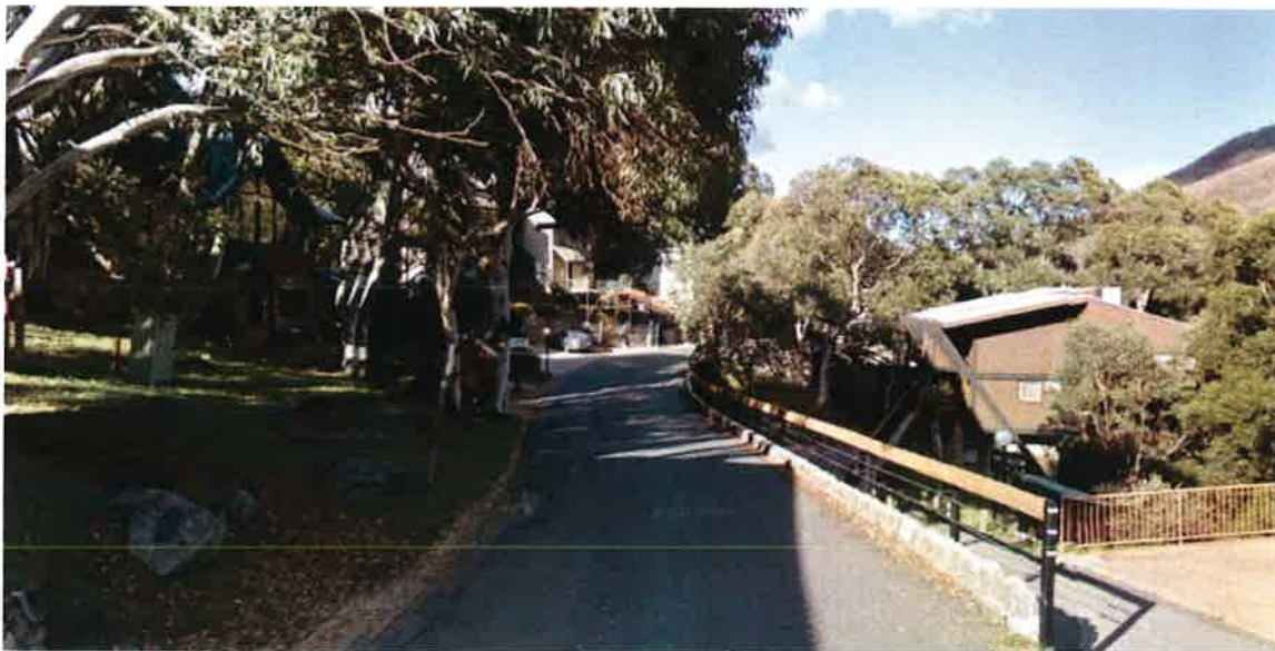
Figure 5 North-West view from Diggings Terrace showing Athol Lodge to the left of image.
